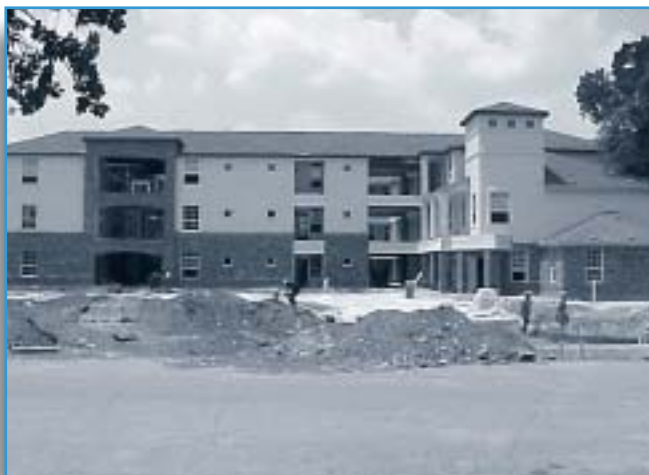
Edwood Place Apartments under construction.
