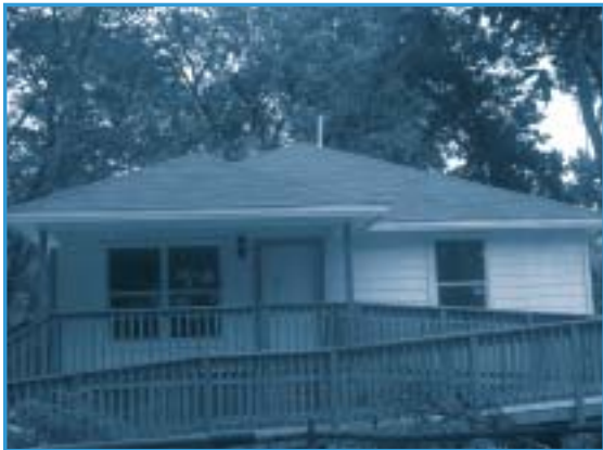
Accessible home rebuilt by GHURC
